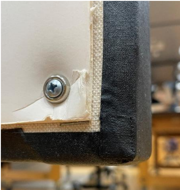
Image 6: Fill on the bottom, left corner (lower right as seen from back), where the tape has fallen away
